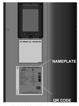
Figure 1. Model and Serial Number Location
